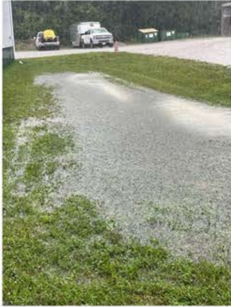
Water ponding outside building
