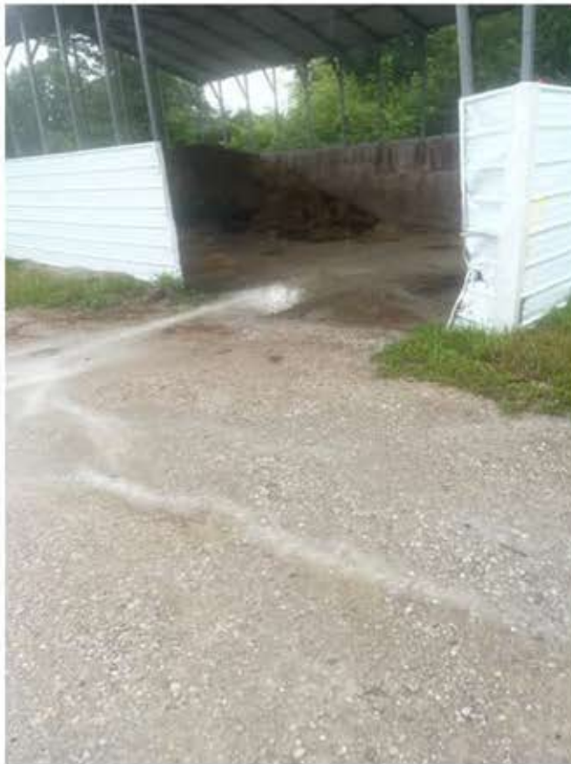
Water draining towards manure shed
