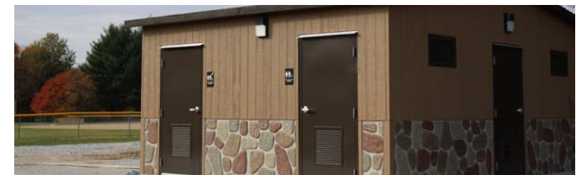
The new showerhouse near the Yellow Banks Park ballfields is ready to greet campers and park visitors for the 2022 season.
